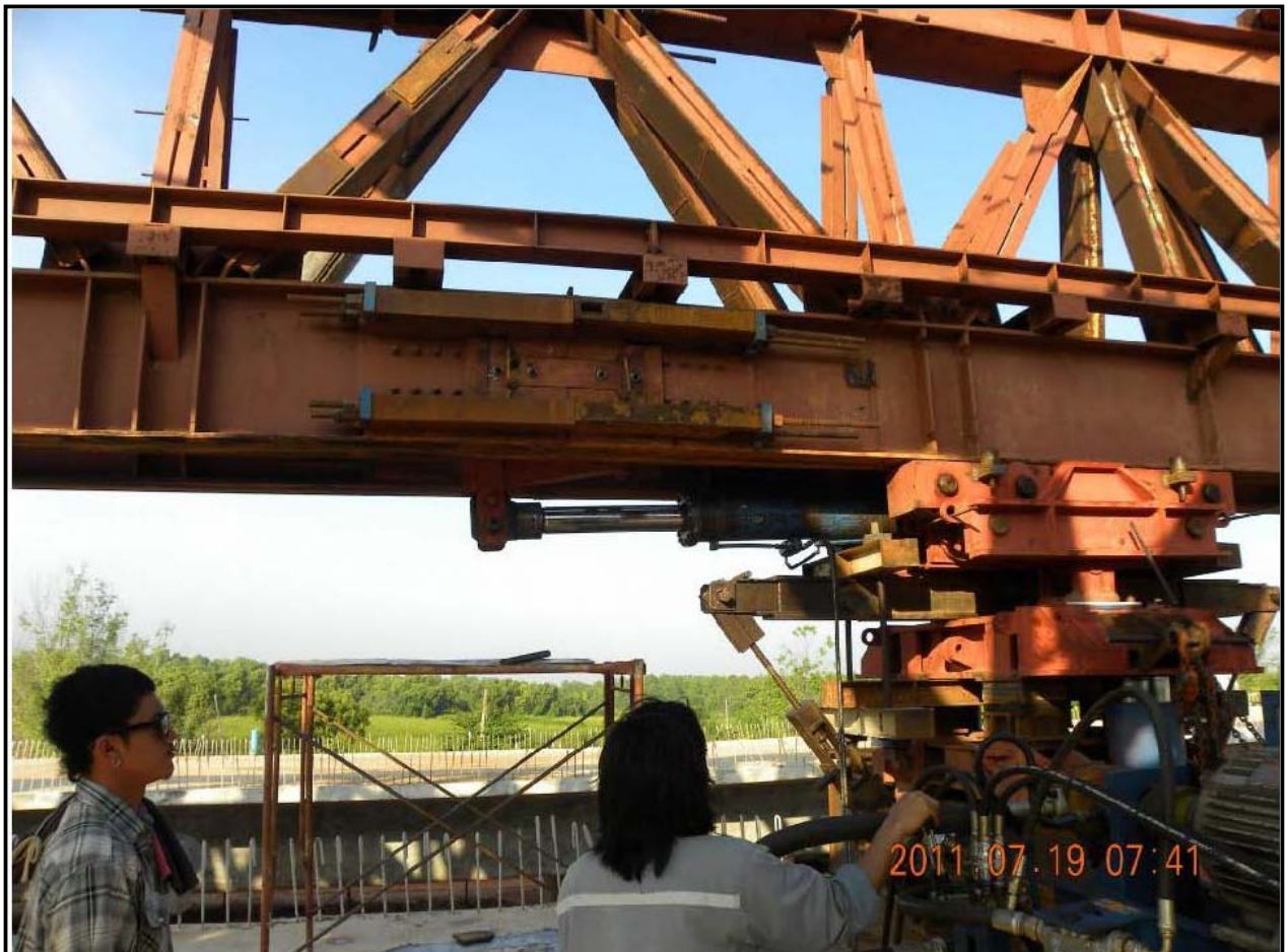
Scaffolding For Super Structure Viaduct(Luanching Truss,Cast In Place)
