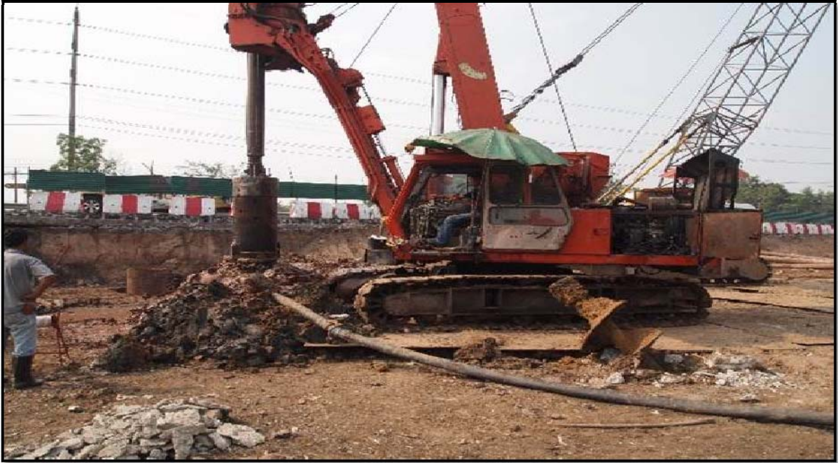
Drilling Crawler Crane
