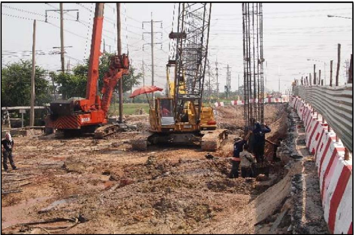
Drilling Crawler Crane
