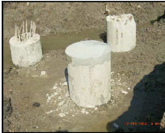
3.3 Static Load Test on Bored Piles
