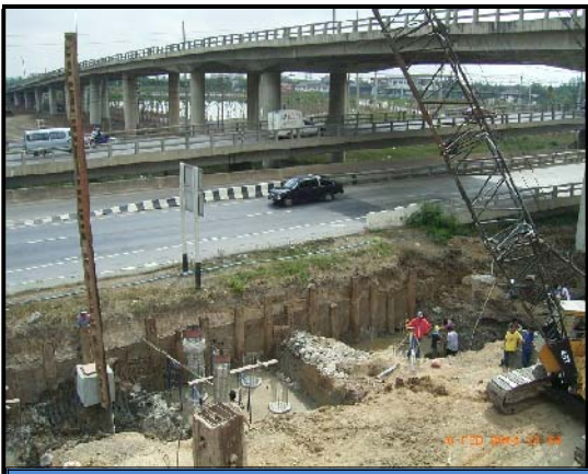
3.4 Dynamic Load Test on Bored Piles
