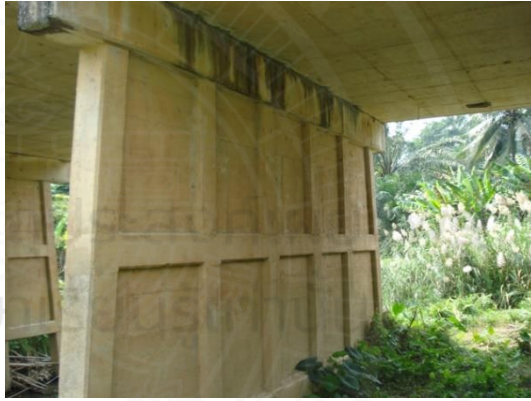
Pile Bent with Wall Bracing
