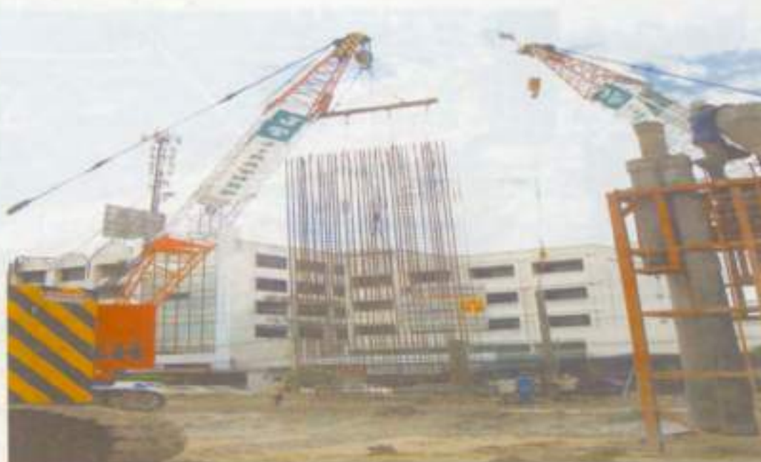
Supports for Reinforcing cage
