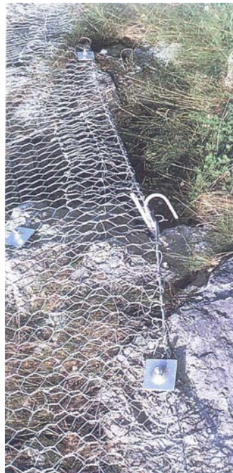
ก) Fissured Hard Rock
